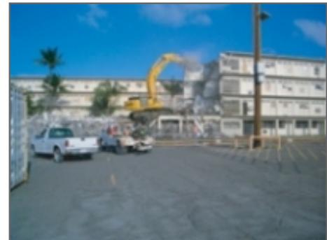
demolishing and downsizing more than 250 buildings (2 million square feet) existing on Johnston Island. Parsons also sorted, transported, placed, and backfilled over all demolition debris on the island and staged recyclable materials for off-island transport.
