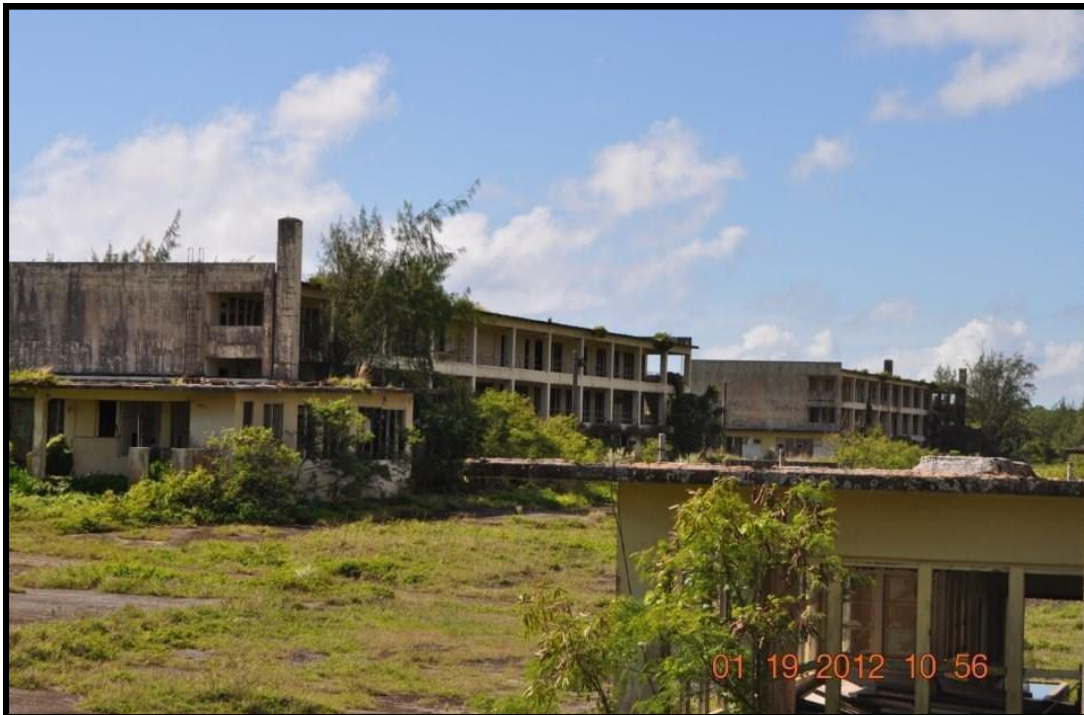
This picture is of the abandon Marbo Barracks as it looks today. They were built “typhoon proof” out of concrete.
